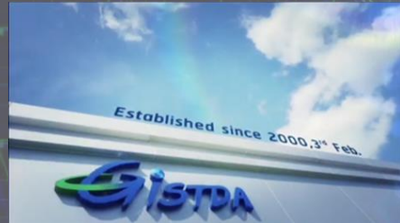
GISTDA Headquarter , Government Complex • Administration • GI Data & Applications Center
